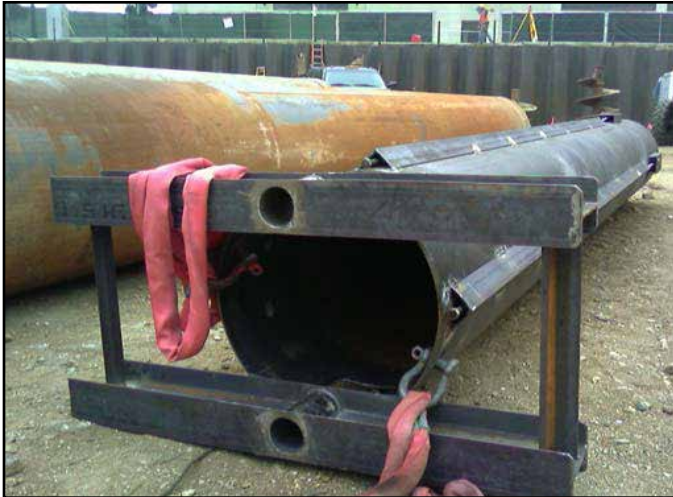
Figure 6: Column installation template
