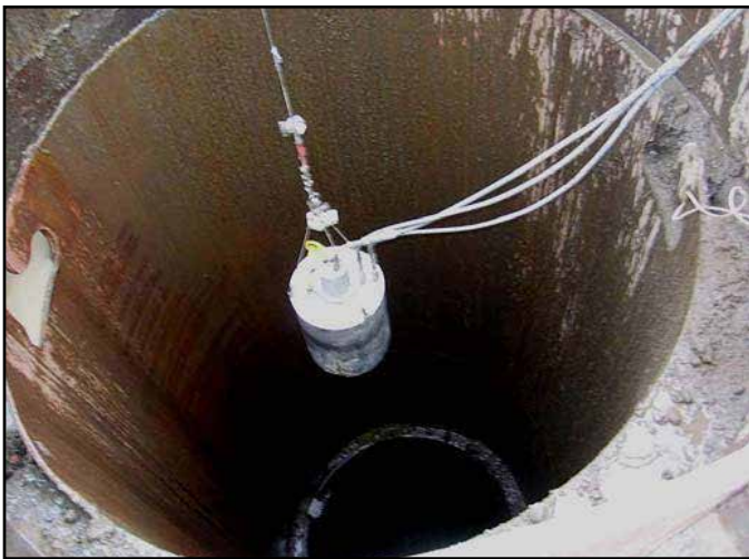
Figure 10: Drilled shaft inspection device
