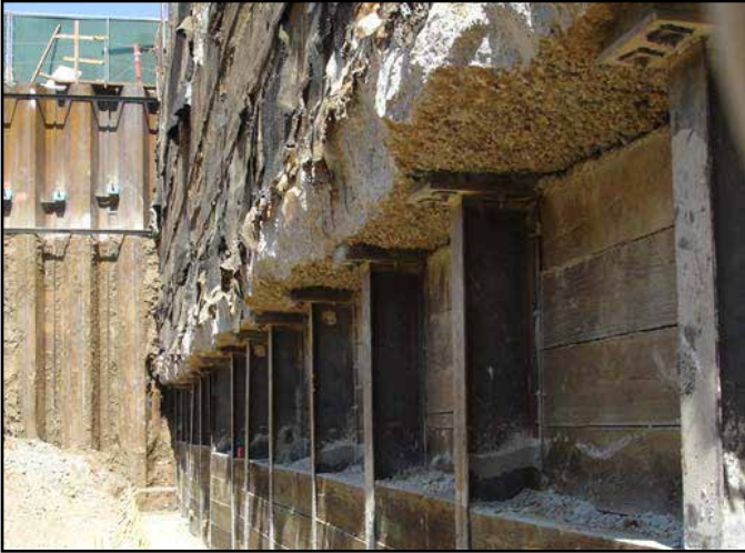
Figure 13: Underpinning at existing DWP vault
