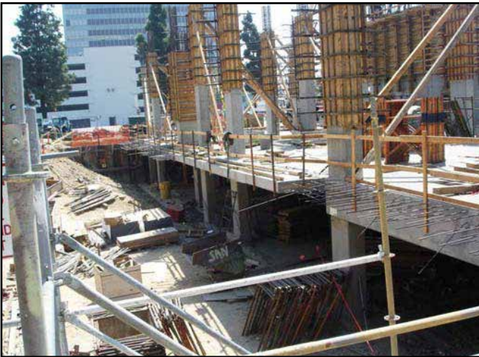
Figure 4: P1 slab in place, construction proceeds upward in up-down zone
