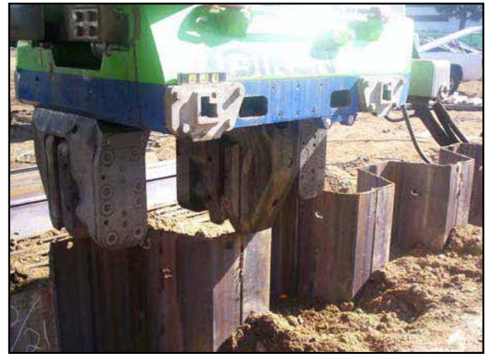
Figure 2: Installation of sheet piles
