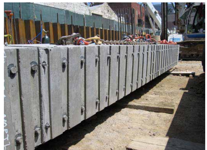
Figure 8: Precast shear wall core corner prior to installation
