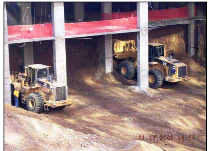
Figure 5: Mining excavation beneath P1 slab
