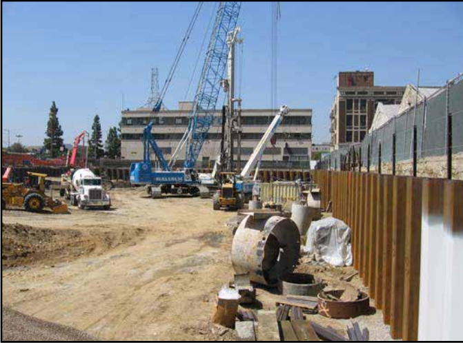
Figure 3: Excavation to P1 level
