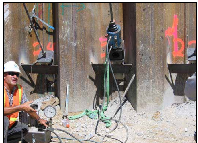
Figure 12: Installation and tensioning of tiebacks at sheet pile within conventional zone
