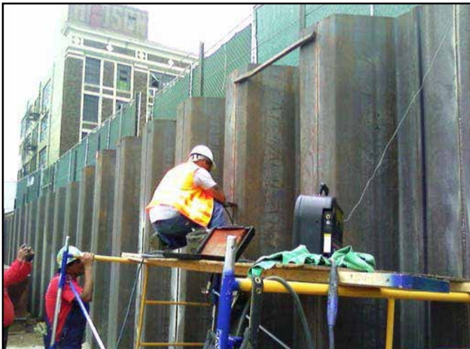
Figure 9: Magnetic particle testing following welding of sheet pile
