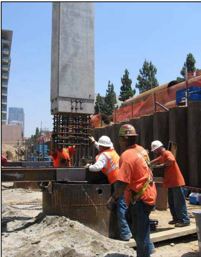
Figure 7: Lowering precast gravity column into place
